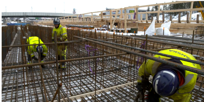
Figure 1: Manual reinforcement installation in progress.
